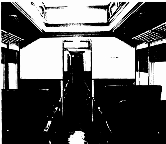
Segregation existed on American Railroads from the 1830s through the 1960s. While states could not impose segregation, private individuals including corporations, like railroad companies, were free to do so. Many railroads used a wall to divide colored passengers from the whites. Noticed the sign to the right that clearly labels the colored compartment.
