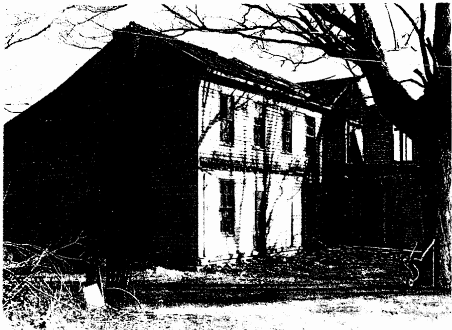
Old Plantation Home of David Richards while being demolished by Bert and Dennis Jolly in the 1980s.
